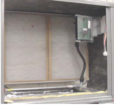
Fig. 22 - Return Air Sensor Operating Position
